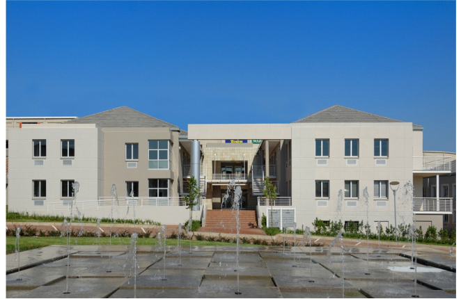
The attractive Greenstone Hill Office Park
