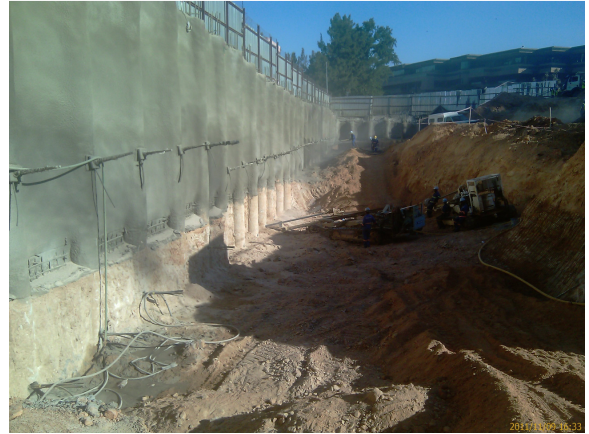
KATHERINE & WEST EARTHWORKS UNDER WAY
