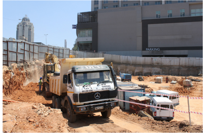
CONSTRUCTION OF KATHERINE & WEST HAS BEGUN
